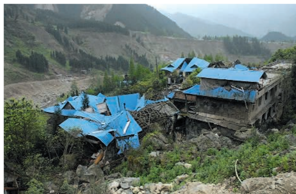
End of the line. The road to Baishuihe disappears just past this wrecked hotel in Longmenshan town.
